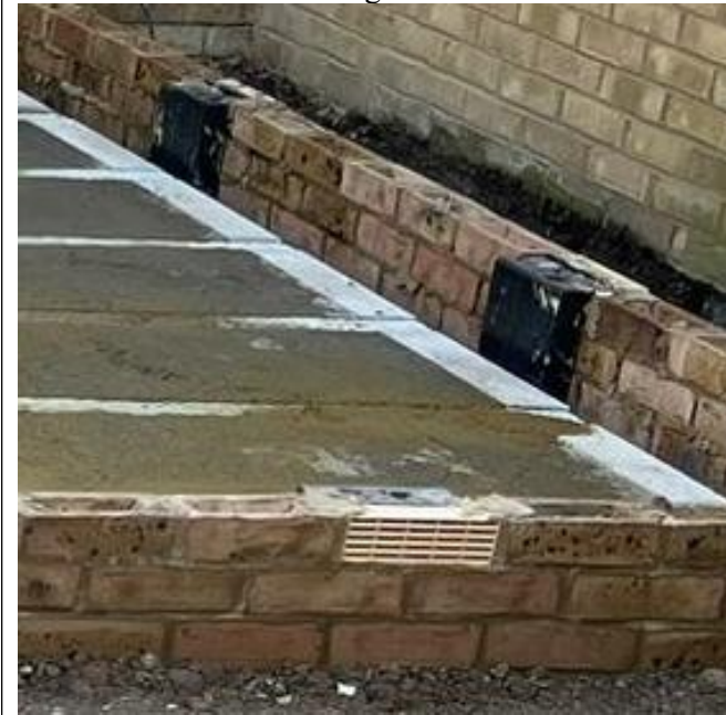
The new extension showing the ventilation next to the garden and the party wall line
