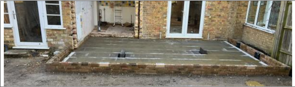
The new extension showing the ventilation next to the garden and the party wall line
